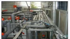
Recovery of cooling water from electronics manufacturing factory by EDR process (Tiger company) (550 m<sup>3</sup>/day)
