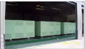
Desalination and reuse of wastewater from precious screw manufacturing factory by EDR process (Nitto company, 350 m<sup>3</sup>/day)
