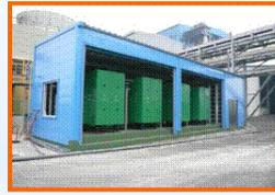
Recovery of wastewater from chemical company for cooling water by EDR process (800 m<sup>3</sup>/day)
