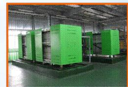
Recovery of wastewater from nylon fiber manufacturing company for cooling water by EDR process ( 800 m<sup>3</sup>/day)
